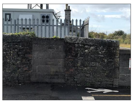
Plate 12. 21: Blocked pedestrian entrance to Buttevant Station (AH020), XC219
