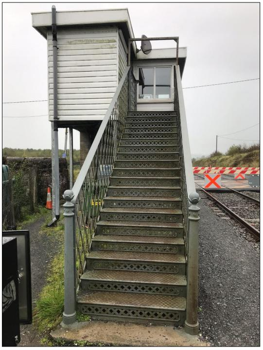
Plate 12. 22: Former footbridge, reused as steps to gatekeeper's hut, XC219 Buttevant (AH020), XC219
